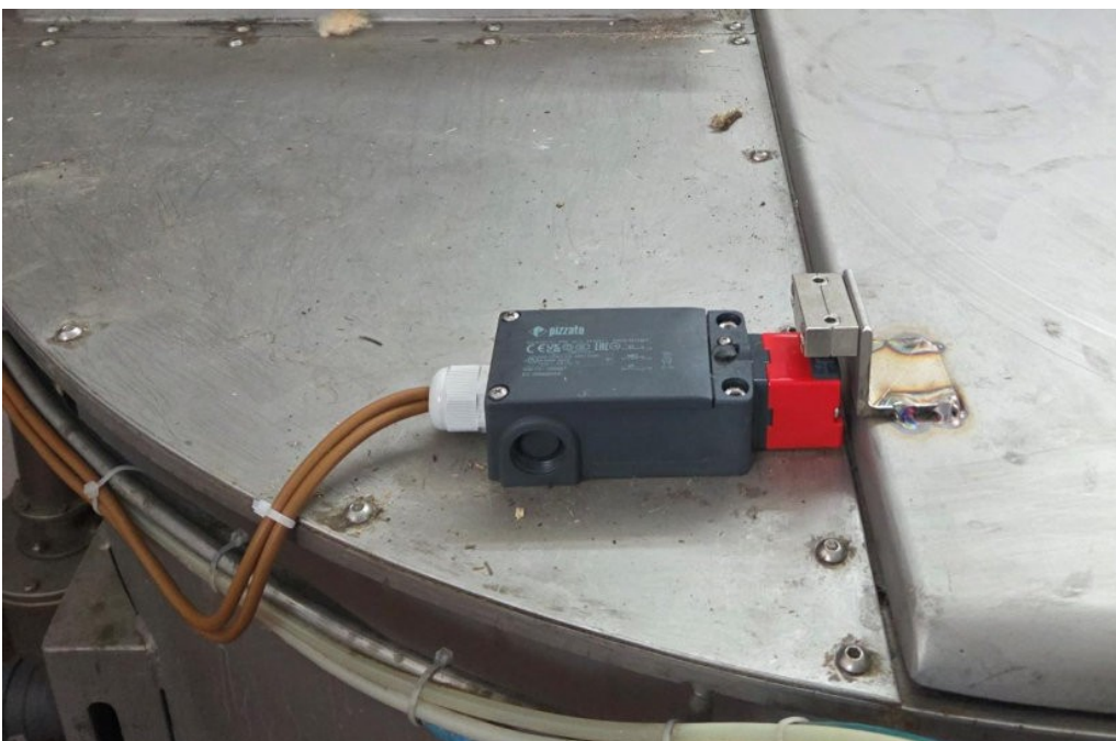
Figure 15 - Detail of safety lock on left-hand door
