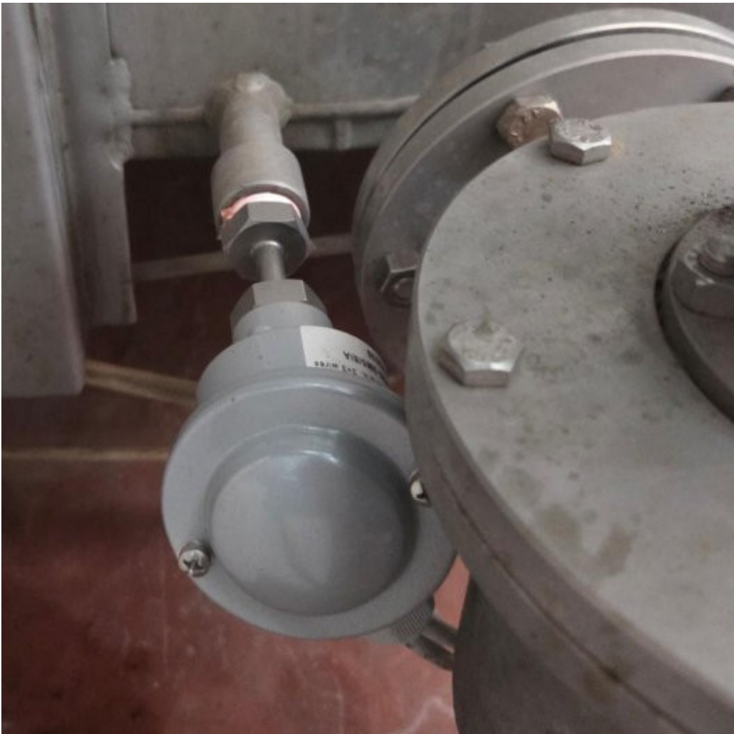
Figure 9 - Detail of temperature probe
