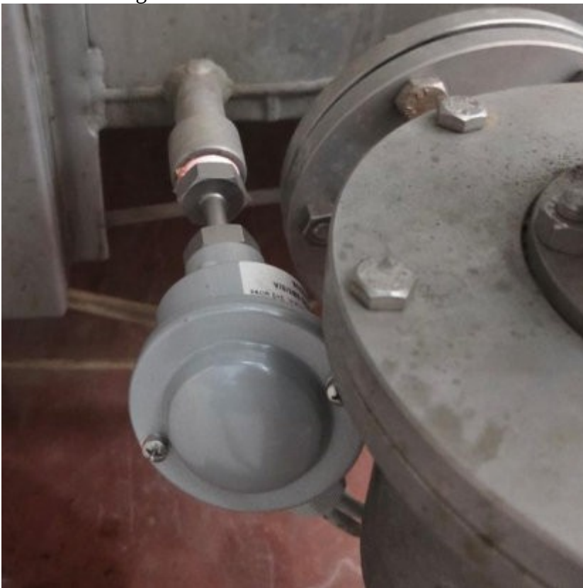
Figure 11 - PT100 probe
